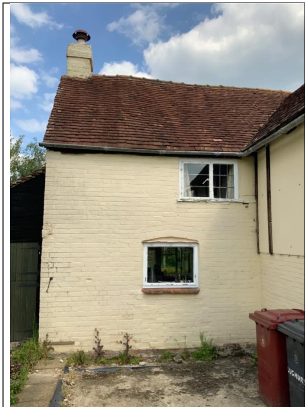
Figure 16, West Elevation of main range. Author 2019.
