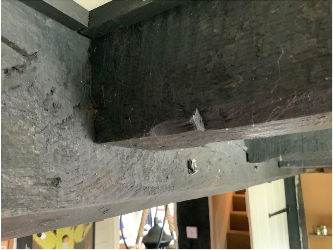
Figure 3, Showing "Lamb's Tongue" chamfer stops on joists. (by Author 2019).
