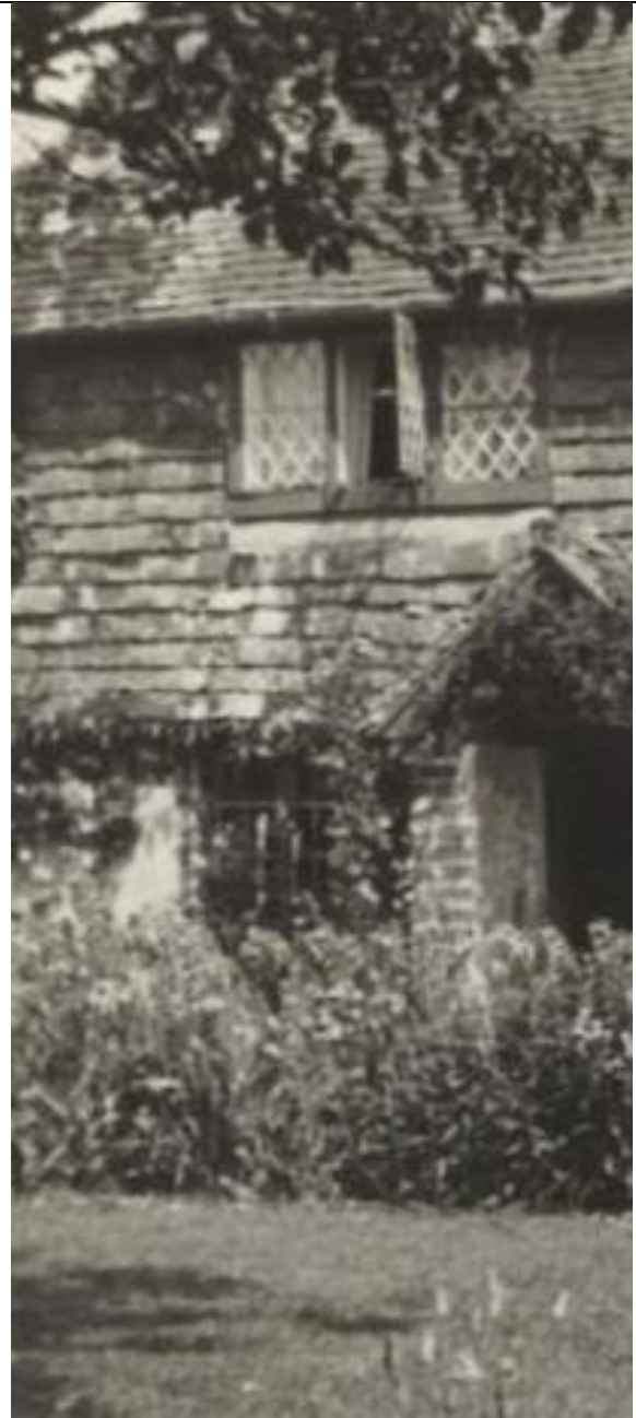
Figure 10, 1937 Photograph of the same windows.
