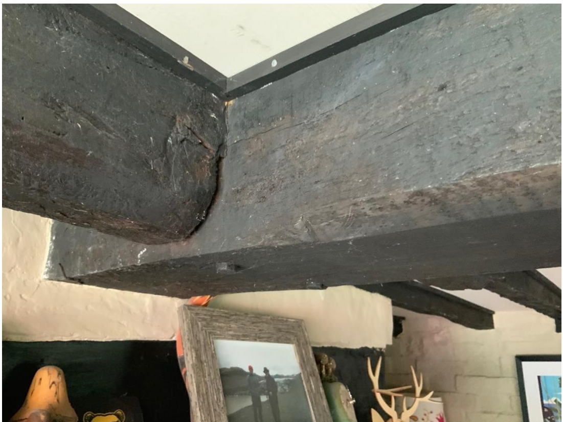
Figure 4, Showing chamfer stops on the spine beam (by Author 2019).
