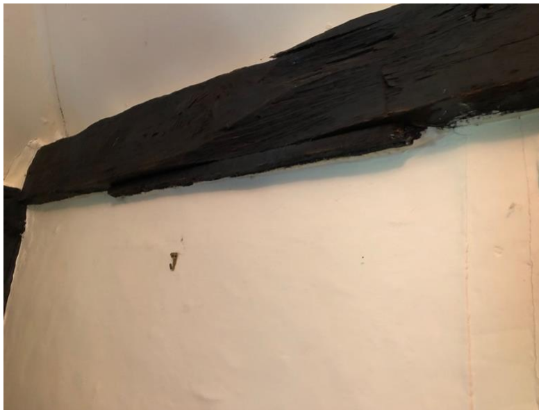
Figure 13, Possible Shutter runner in South elevation, (Author 2019)
