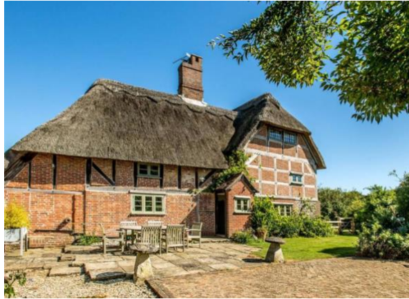
Figure 6, Black House Farm House.
